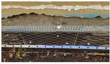
wire mesh, stainless steel weep screed and flashing are installed and readied for inspection by the building inspector.
