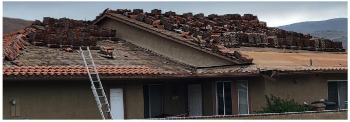
Eventually, a full tile relay (shown in photo above) will be required as part of the standard maintenance cycle for the tile roofs. Several homes in the nearby Yorba Linda area are currently undergoing underlayment, flashing, and tile replacement (if needed). Funding the work is anticipated to provide the greatest challenge to the Association as Construction Cost Inflation is significantly higher than the CPI, PPI, and CPE indexes that residents may be familiar with.
